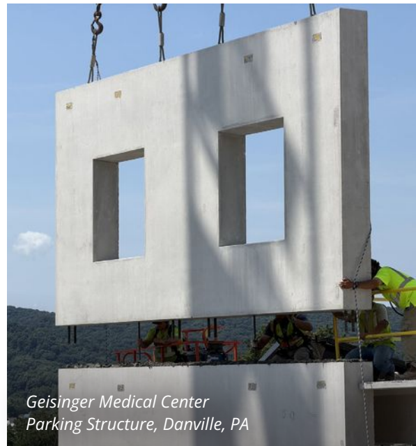
Wall Panel Installation, Leesburg, VA
